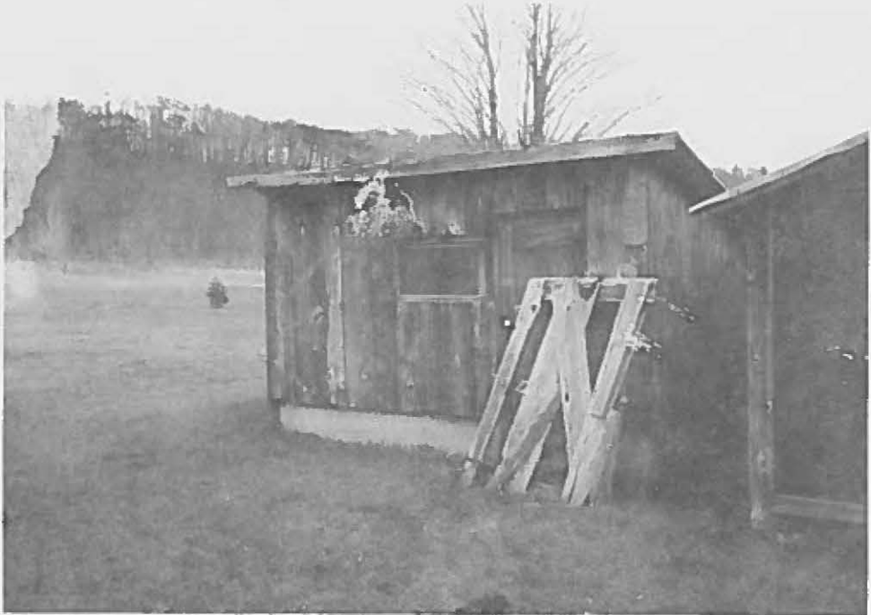
Baur Brooder House (HS 35-118F)
