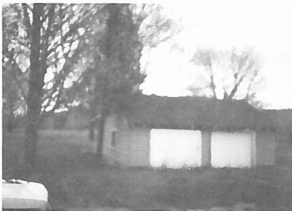
Kelderhouse Garage (HS 35-183B)
