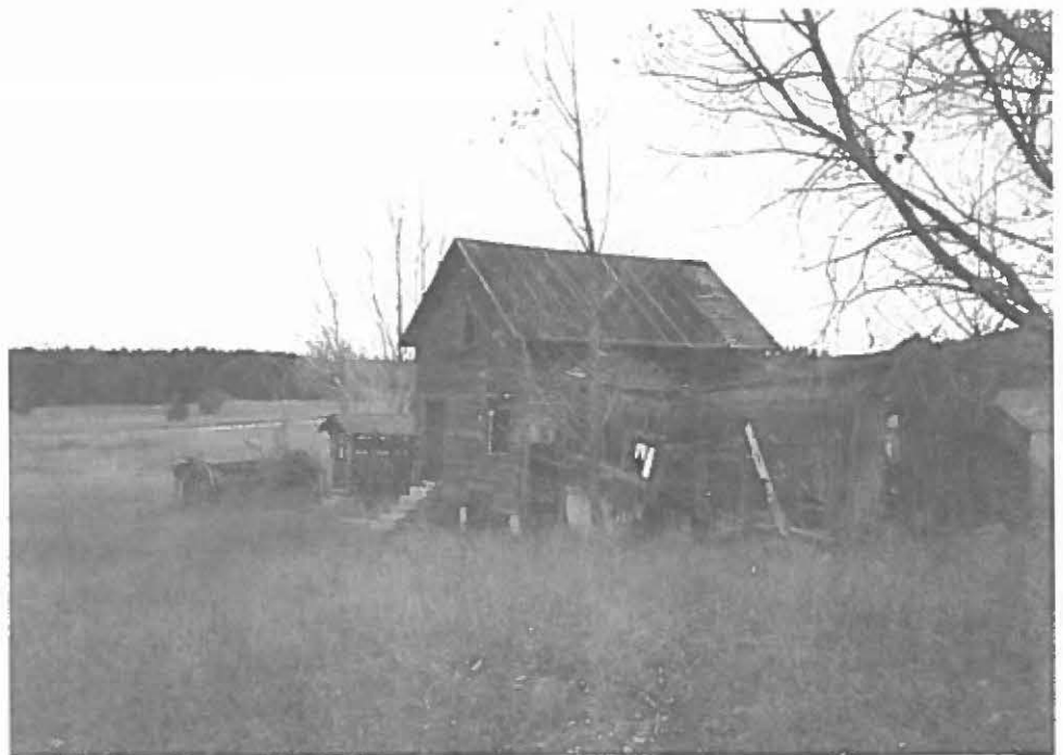
Milton C. Basch Shed #3 (HS 35-199D)
