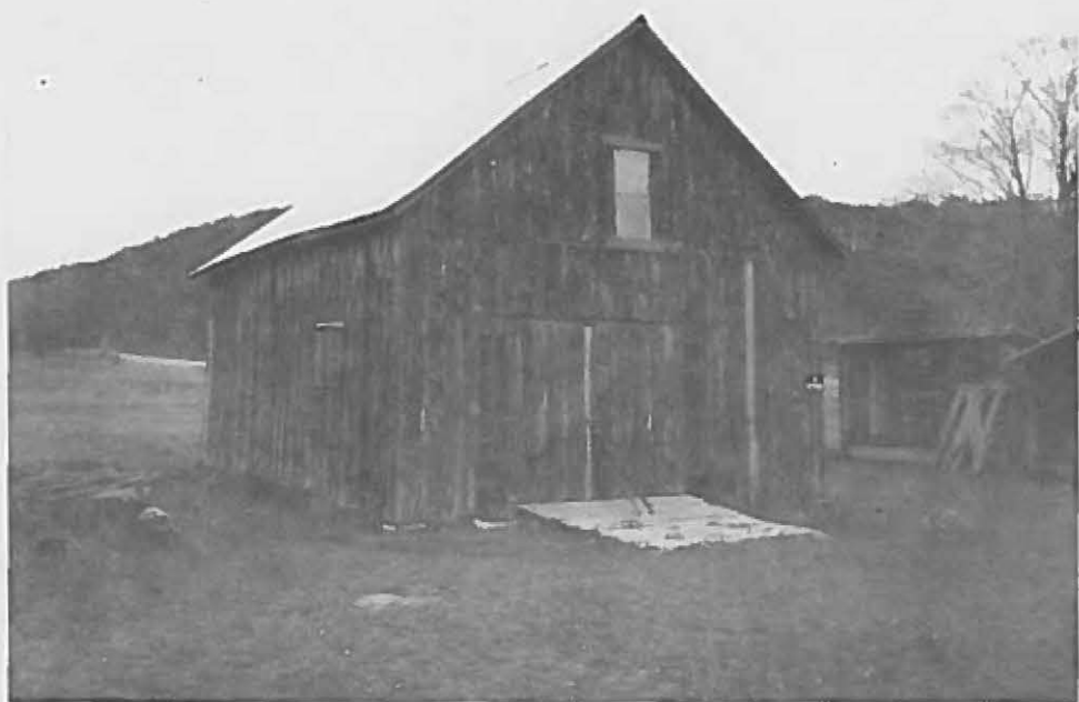
Baur Small Barn (HS 35-118C)
