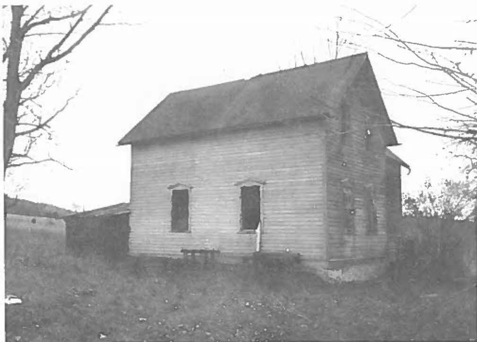
Milton C. Basch House (east) (HS 35-199A)
