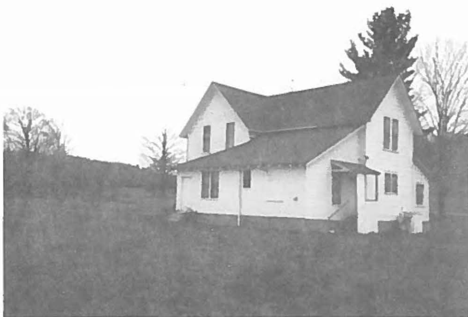
Kelderhouse House (southwest/rear) (HS 35-183A)
