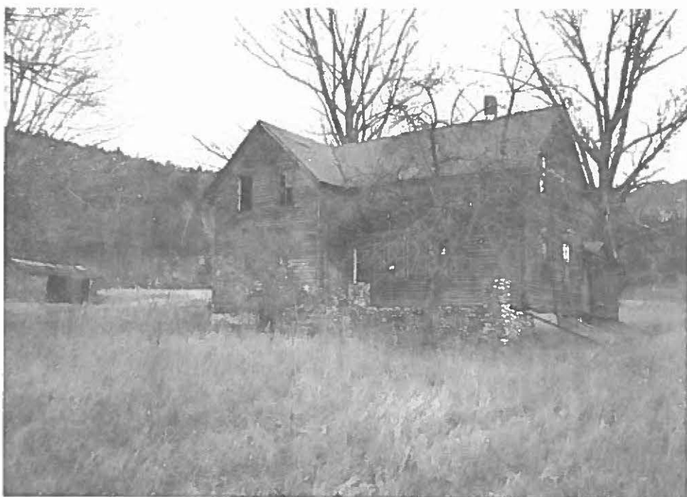
Milton C. Basch House (west) (HS 35-199A)
