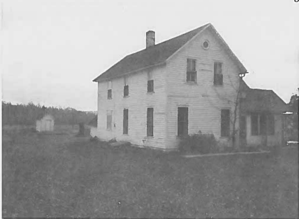
Burfiend House #1 (west/front) (HS 34-139A) and Privy (HS 34-139D)
