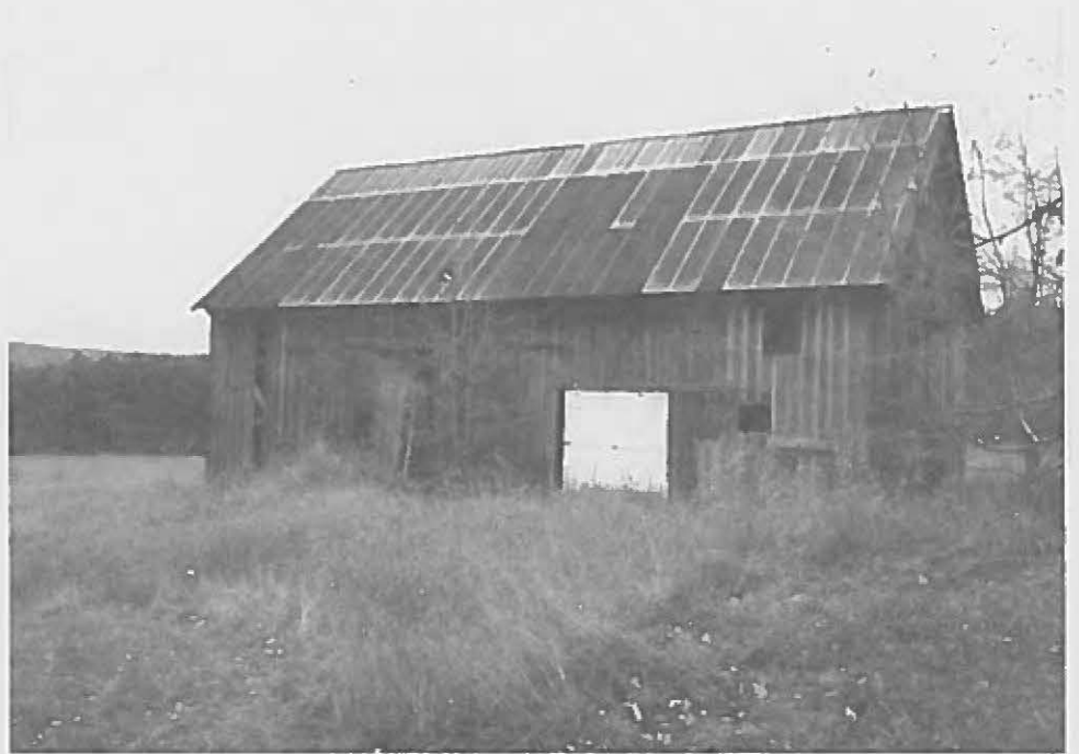
Miller Centennial Barn (HS 34-153)
