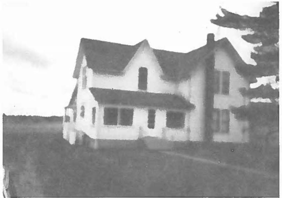
Kelderhouse House (north/front) (HS 35-183A)
