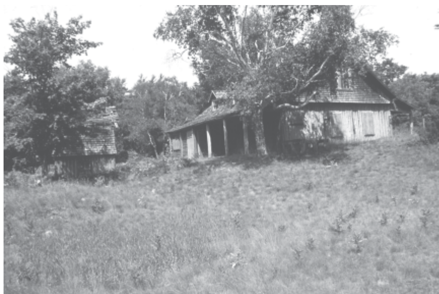
Figure 5.23. Alvar and Mary Bournique residence and ice house, 1996. The complex retains historical integrity, but it is deteriorating rapidly.
