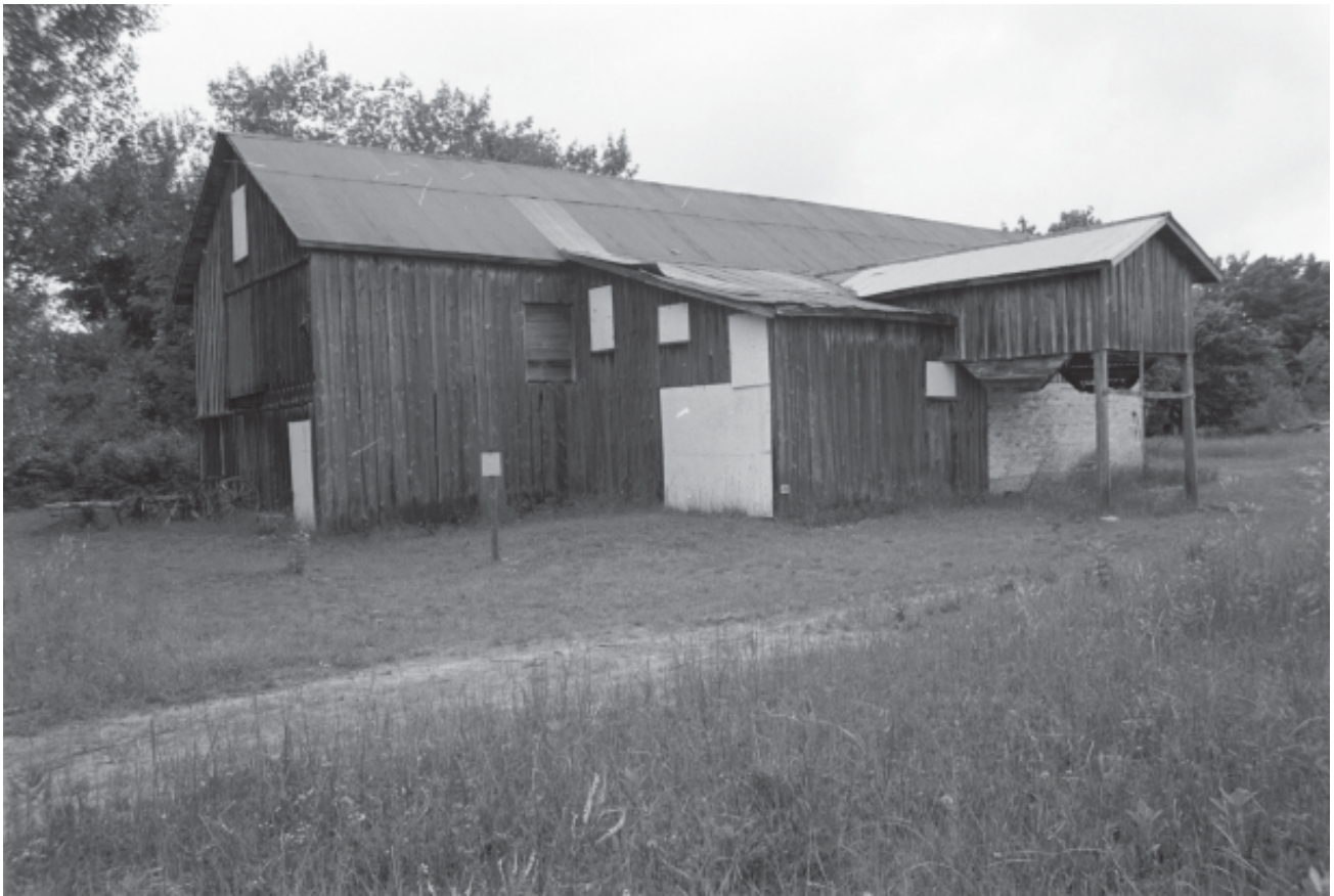
Figure 4.23. Manitou Island Association sawmill, 1996. The mill is partially composed of materials salvaged from Peter Stormer's mill at the southeastern end of the island. The sawmill was not central to the MIA's agricultural operations, but it did produce materials that the association used to construct and maintain its various farm structures. The mill was situated below the beach ridge on a site located several hundred feet from the barn, perhaps to provide ample room for piles of logs and lumber without interfering with nearby farming activities. The MIA sawmill remains in sound structural condition, representing two important phases of twentieth-century logging activity on North Manitou Island.
