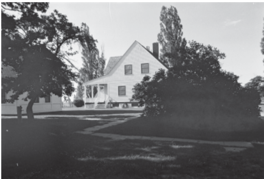
Figure 4.102. U.S. Life Saving Service dwelling and large lilac shrub, 1996. The largest building in the North Manitou USLSS complex, the dwelling was constructed in 1887, and subsequently remodeled by the U.S. Coast Guard during the early 1930s. After a fire destroyed the Manitou Island Association lodge in 1953, the MIA rehabilitated the former USLSS dwelling to house groups of sportsmen who traveled to the island to hunt and fish.
