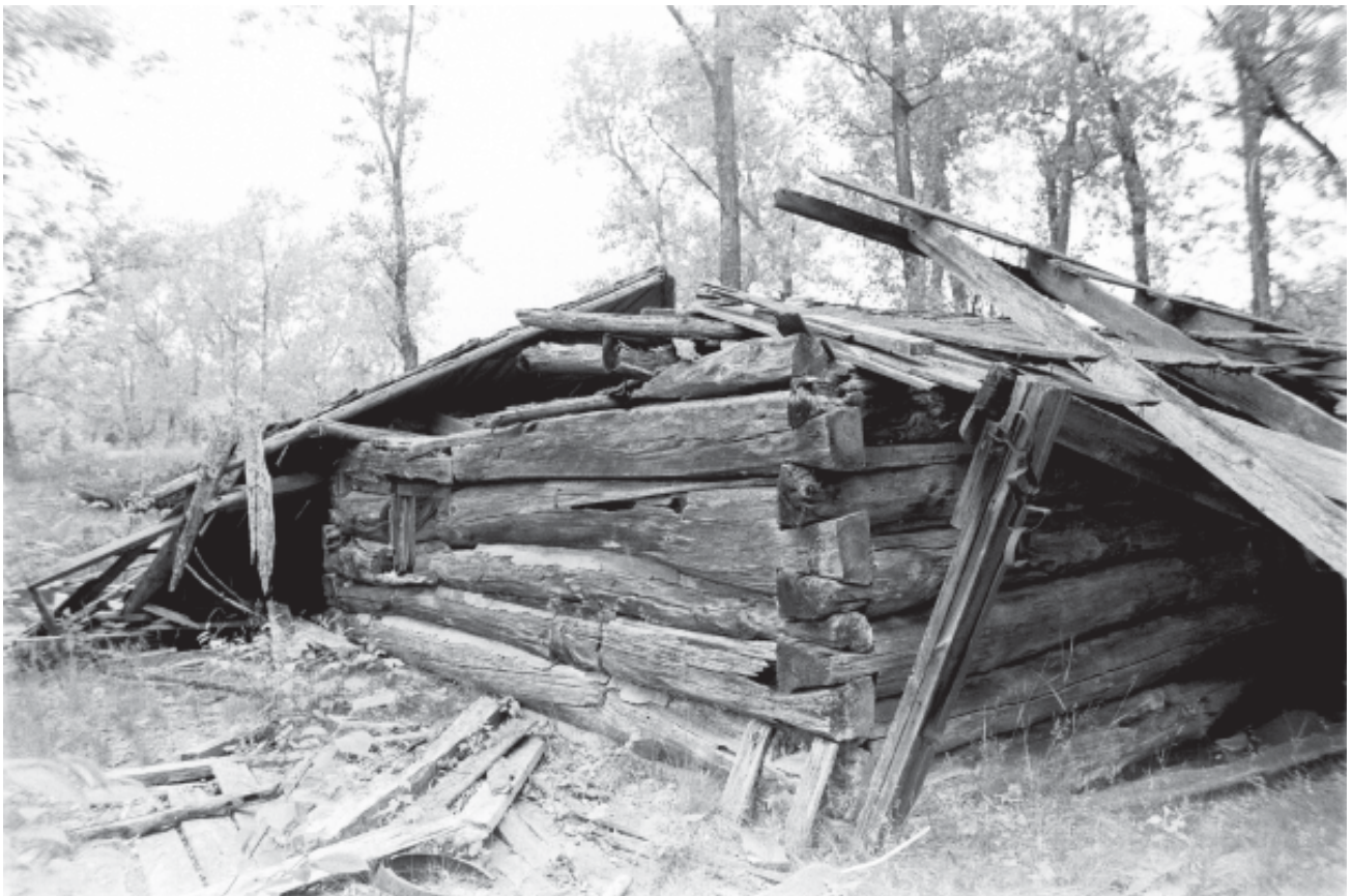
Figure 4.50. Small log barn ruin, Alvar and Mary Bournique farm, 1996. The lower walls of this small barn were constructed of large, hewn timbers with full dovetail corner notching.
