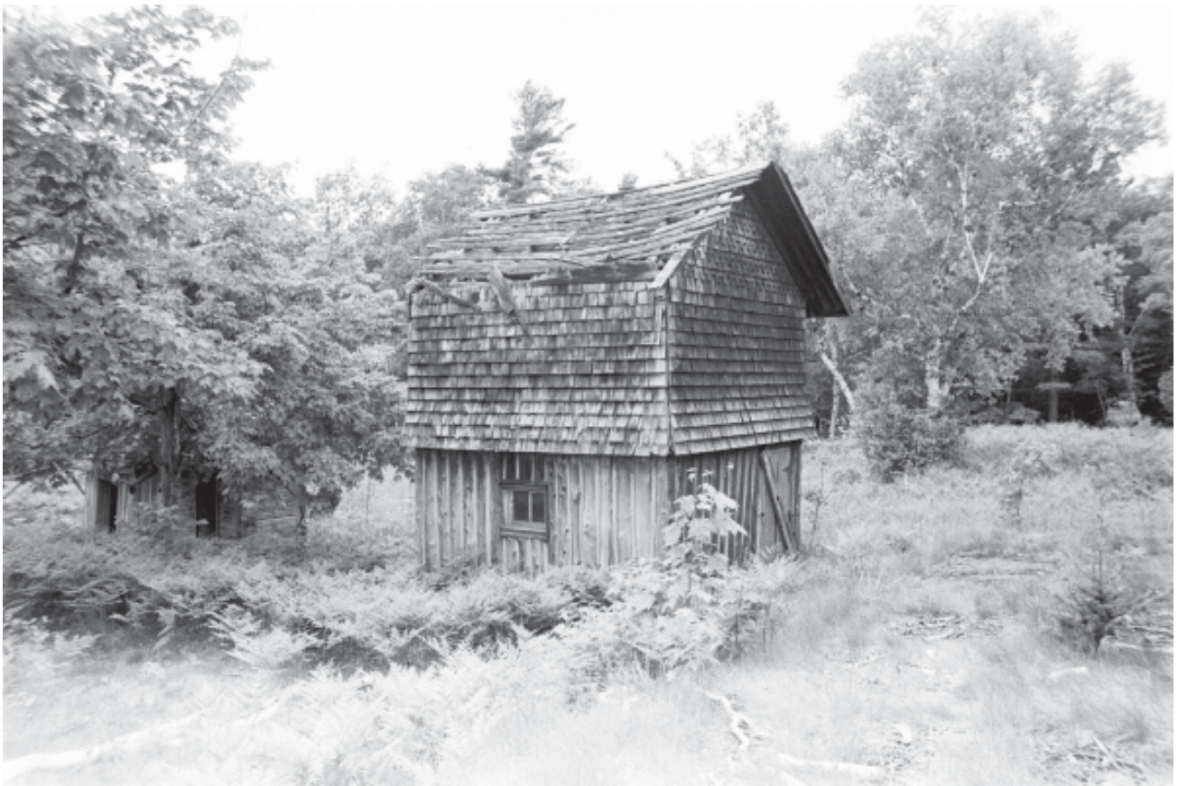
Figure 4.56. Alvar and Mary Bournique ice house, 1996. The Bournique ice house is one of the most visually intriguing structures on North Manitou Island. Its form, decoration, and exterior cladding materials complement the architecture of the residence.
