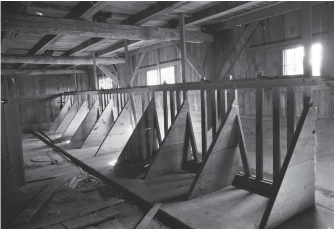
Figure 4.37. Manitou Island Association west-side barn, milking stanchions, 1996. The floor plan, materials, equipment, and interior finishes of the MIA barn conform to standards promulgated during the 1910s and 1920s by the U.S. Department of Agriculture and the extension programs of state agricultural colleges.
