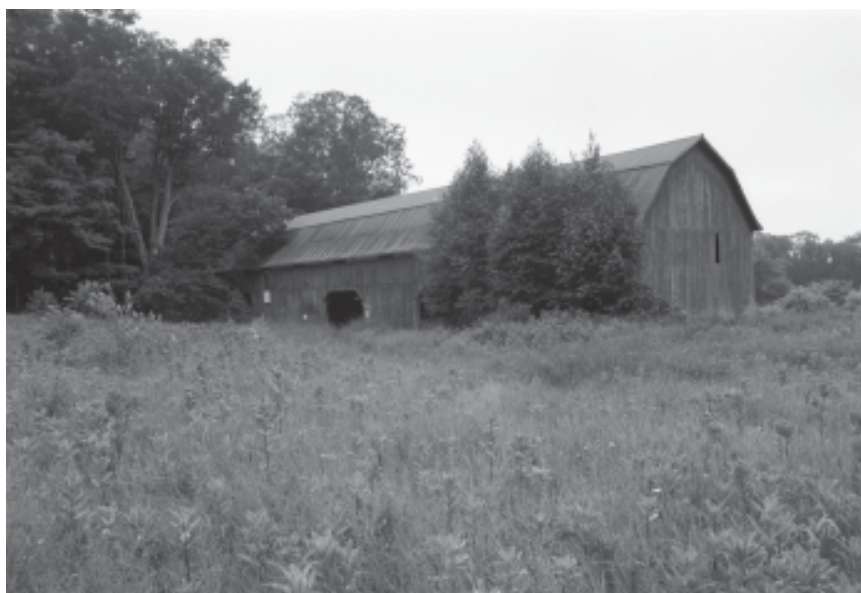
Figure 4.35. Manitou Island Association west-side barn, eastern and southern facades, 1996. The barn is a prominent landscape feature of the west-side farm clearing and Crescent townsite, and dramatically frames westward views of Lake Michigan.
