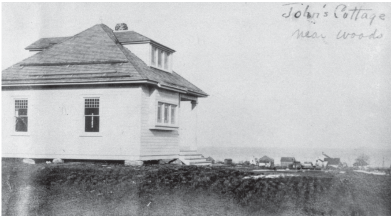
Figure 4.130. The cottage built for John Newhall near the edge of the North Manitou Village clearing, ca. 1900. The cottage served as Newhall's residence while he was on the island managing the family's extensive agricultural and resort business.
