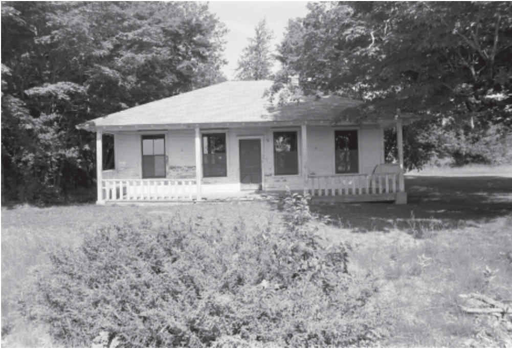
Figure 4.117. Frederick H. and Mary Trude cottage, front (eastern) elevation, 1996. The Trude cottage is one of three Cottage Row houses that appear to be influenced by vernacular dog-trot bungalows, a common house type in Gulf Coast resort communities. The broad front gallery of the Trude cottage takes advantage of the building's orientation toward the Manitou Passage.
