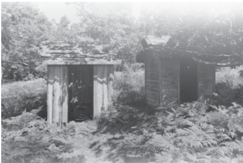
Figure 4.57. Alvar and Mary Bournique privies, 1996. Privies of two different designs line the walkway that leads downhill from the terrace behind the Bournique residence. One of the privies, clad with vertical logs, evidently was designed to match the architecture of the residence and ice house.
