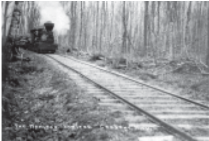
Figure 2.19. Smith & Hull narrow-gauge railroad, near Crescent. A 28-ton Shea steam engine hauled timber along a six-mile rail spur which extended from the interior of the island to the lumber mill and dock at Crescent.
