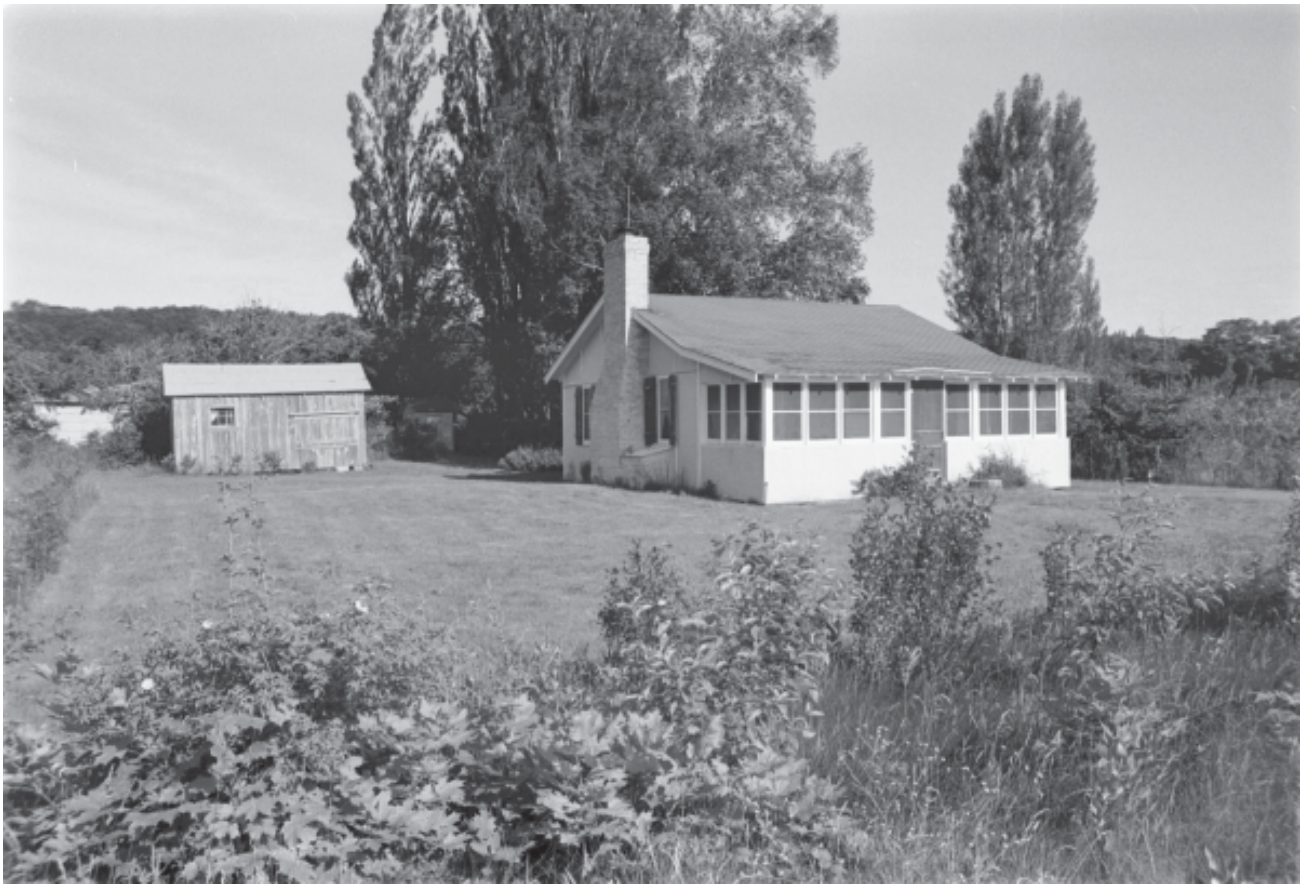
Figure 4.126. Shirley Foote Alford cottage and migrant orchard workers' cabin, 1996. A "mail-order" house, the Alford cottage represents a practical solution to the dilemma of constructing a building in a remote setting that, during the late 1930s, lacked both modern materials and a skilled labor force.
