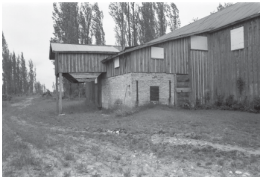
Figure 5.13. The MIA sawmill represents an important theme in North Manitou Island's human history, and is a rare, intact example of a steam-powered lumber mill in Michigan.
