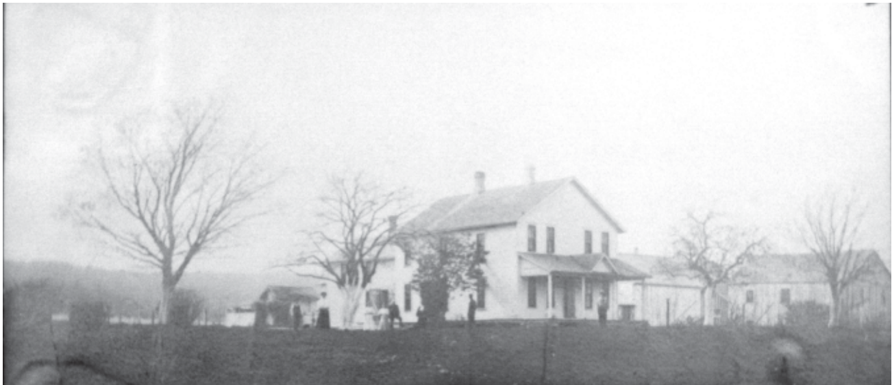
Figure 4.4. The “farmhouse,” ca. 1910s. This structure served as the Boardman family’s North Manitou home. The house subsequently was owned by the Newhall family, the Manitou Island Syndicate, and the Manitou Island Association. It was destroyed by fire sometime in the late 1920s.
