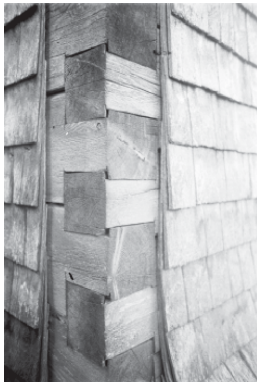
Figure 4.78. Corner notching detail, Lars Christian Alstrom / Peter Stormer house ruin, 1996. Although the Peter Stormer family abandoned the house more than seventy years ago, all four of its side walls remain standing and remarkably intact. Such longevity attests to the durability of the solid corner-joints and exquisite craftsmanship that are evident in the wall construction.
