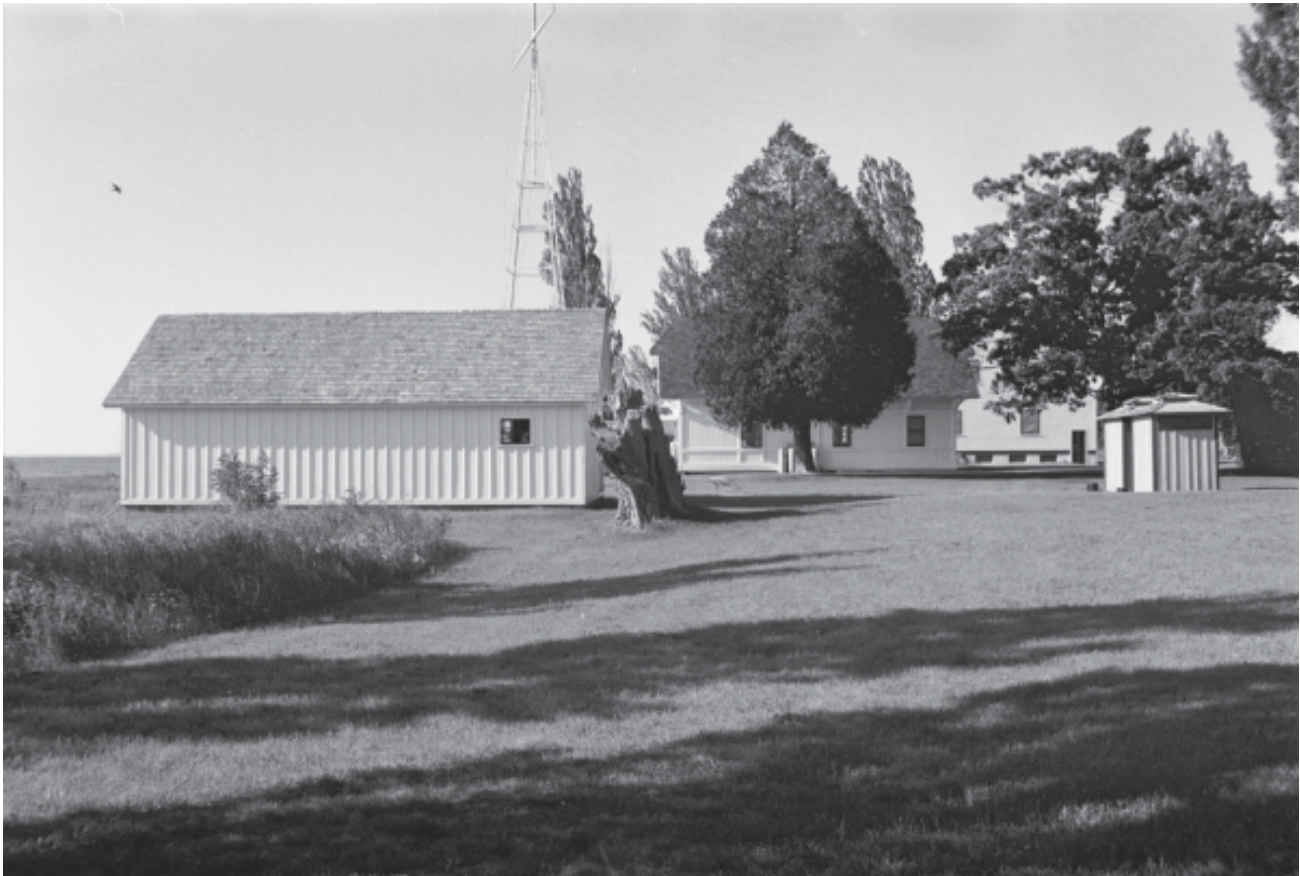
Figure 4.101. 1854 Volunteer Rescue Station beach cart house, north elevation, 1996. This structure dates from the founding of the North Manitou Island volunteer rescue station in 1854. The design of the beach cart house appears to be based on standard plans developed for a series of 28 stations established by the U.S. Secretary of the Treasury under a special 1854 appropriation. It is the oldest structure associated with the USLSS on the Great Lakes.
