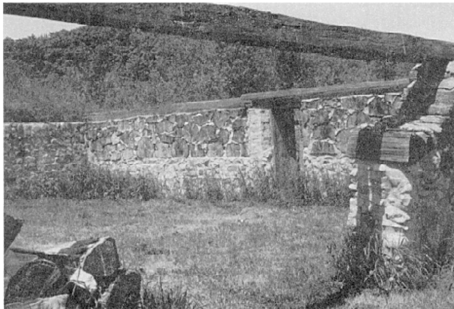
Figure 59. Stovewood Barn Foundation (1994)
