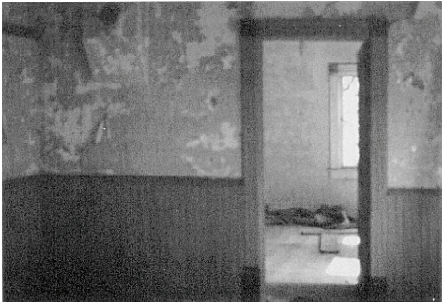
Figure 69. Interior of Farmhouse (1994)
