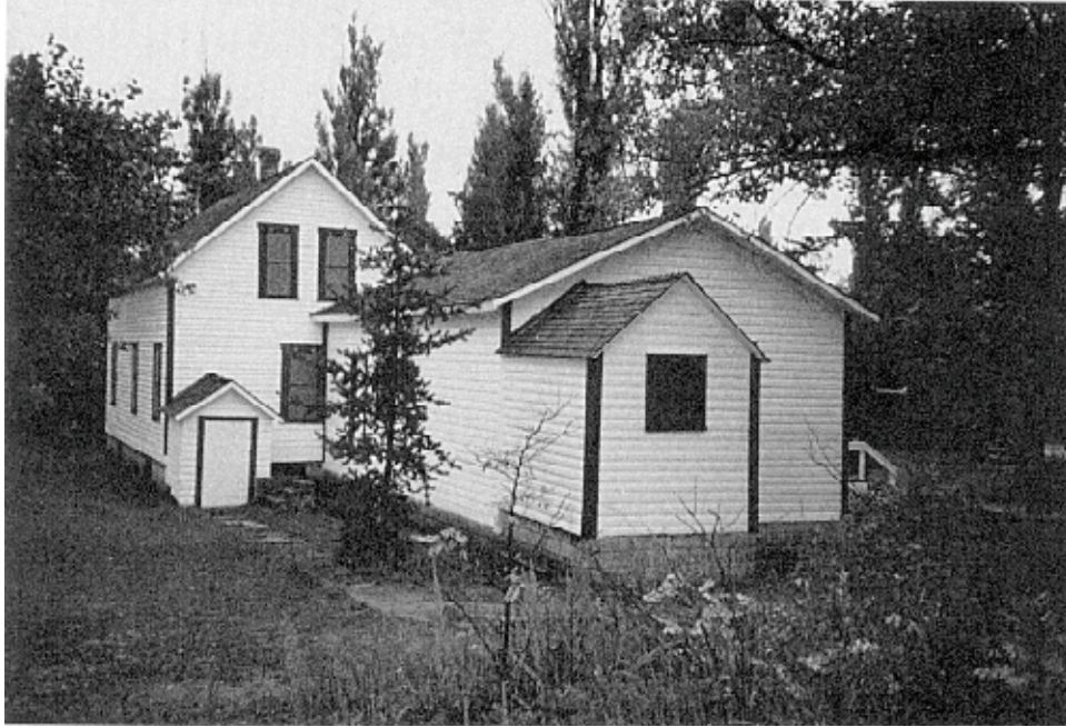
Figure 25. SMI Post Office/Visitor Center Building (1994)
